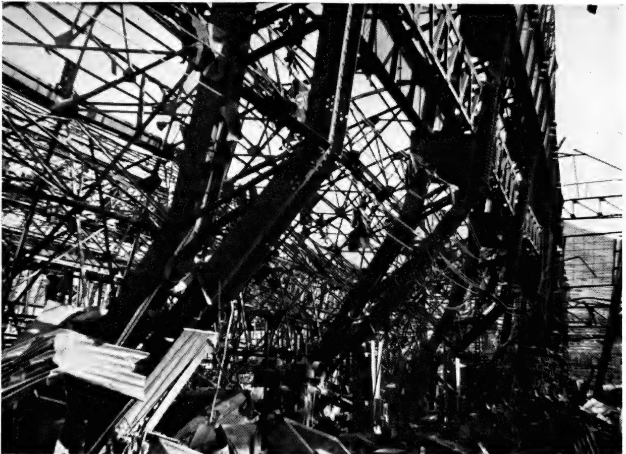
Photo No. 12. NAGASAKI. Large steel framed shed in the Mitsubishi Steel Works, \frac{3}{4} mile from the centre of damage. The steel stanchions have been bent (away from the explosion) and the roof trusses on both sides of these stanchions have collapsed. See paragraphs 22 and 32.
